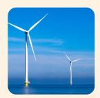
62 wind turbines spaced 1 nautical mile apart with each turbine generating 13 MW of electricity
