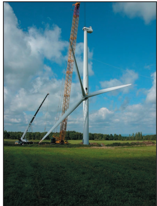
Mounting Rotor to Tower
