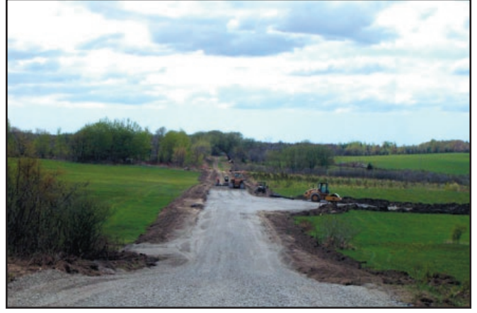
Local and Access Road Upgrades
