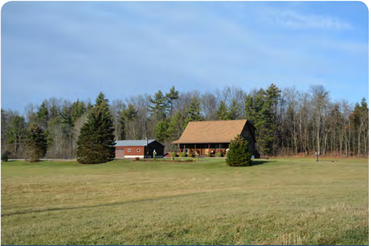
Context Photo: View to the North
