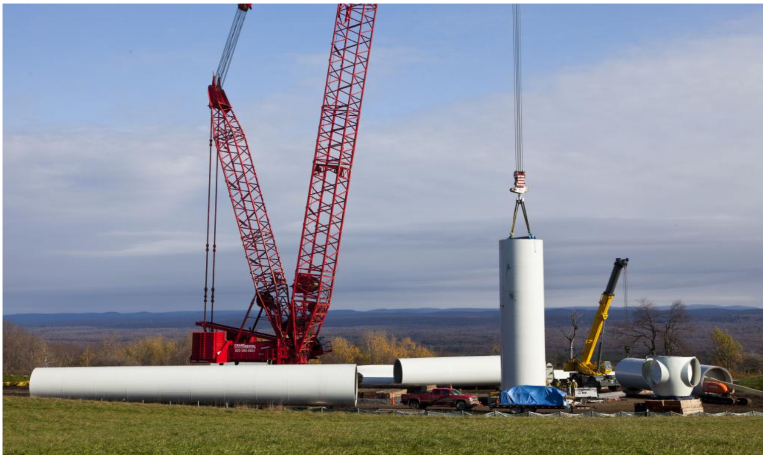
Tower Erection
