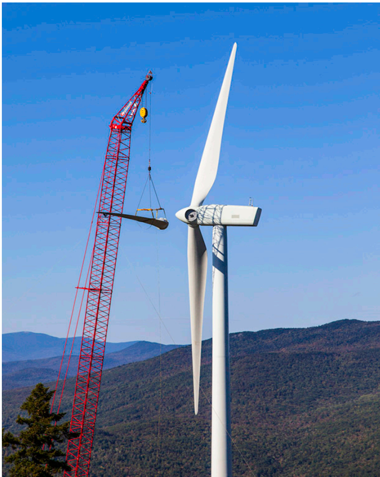
Blade Installation
