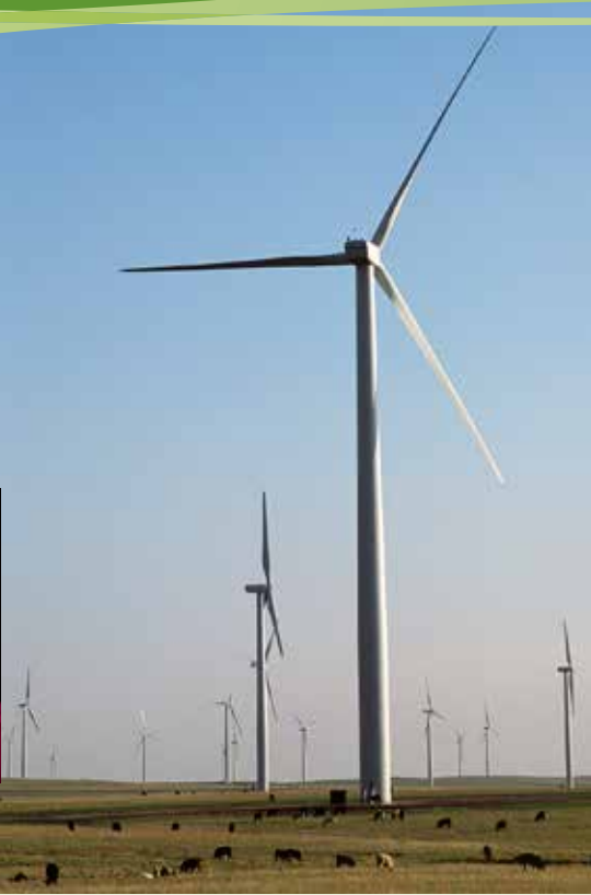
Above: The 150 MW Elk River Wind Project
