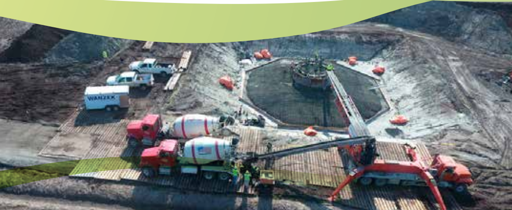
An overhead drone photograph of a wind turbine foundation under construction.
