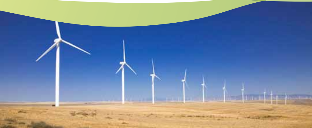
The Hay Canyon Wind Power Project in Oregon features 48 turbines to produce 101 MW of clean, renewable energy.
