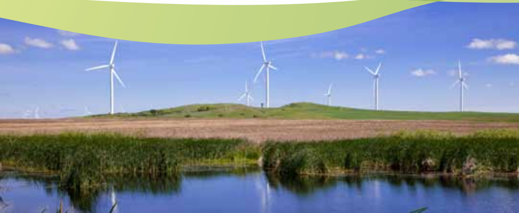
The Rugby Wind Power Project in North Dakota features 71 Suzlon S88 – 2.1 MW turbines to produce 149.1 MW of clean, renewable energy.
