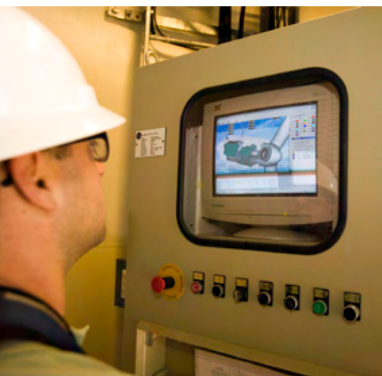
New wind turbines usually require software updates during the first year of operation to account for elevation, terrain and weather conditions.
