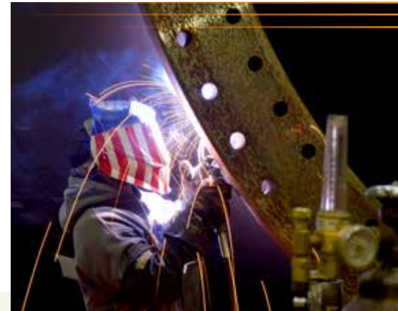
Photo courtesy of Greg Alvarez, AWEA, at Broadwind Towers, Manitowoc, Wisconsin
